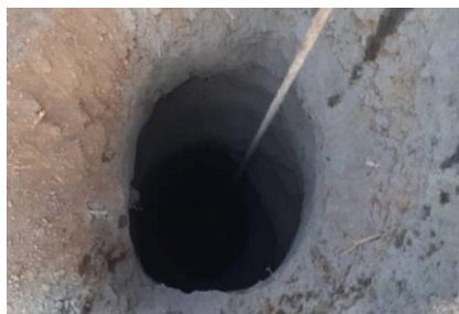
Abandoned bore well being filled with sand, boulders, pebbles from bottom till ground
