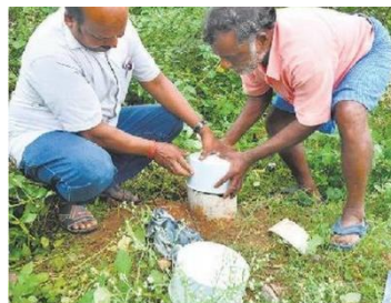
Abandoned bore well being filled with sand, boulders, pebbles from bottom till ground
